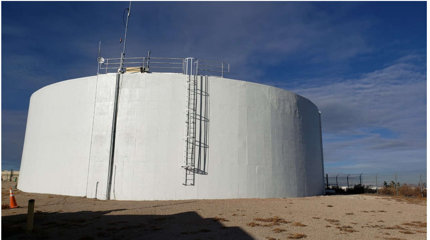
Above is the 1MG Tank repainted in 2022
