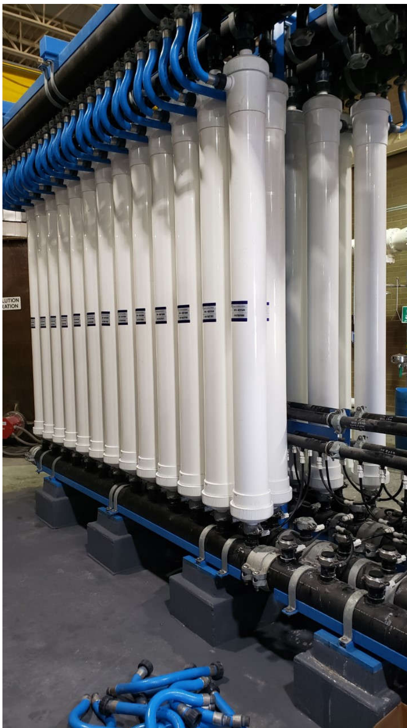
New membranes replaced at the JWPP in 2022
