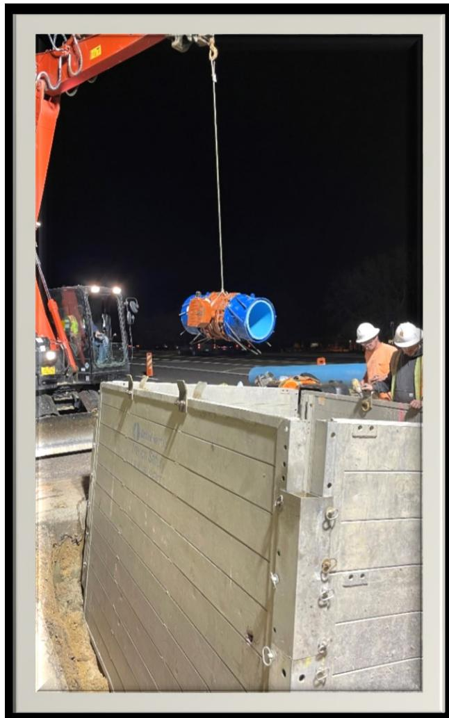
The valve identified with the highest risk of failure was replaced on November 6, 2021, located at the southwest corner of Arapahoe Road and Revere Parkway. This valve has been in service for more than 40 years, and is crucial in maintaining potable water service to customers west of Revere Parkway on Arapahoe Road. This 18" valve wouldn't isolate, which would have caused major issues if there was a water main break to the west.
