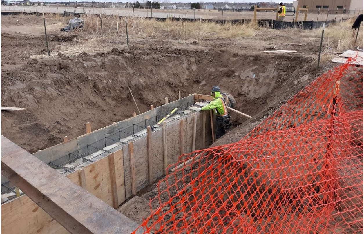
Water Line Encasement at Green Acres Tributary Project
