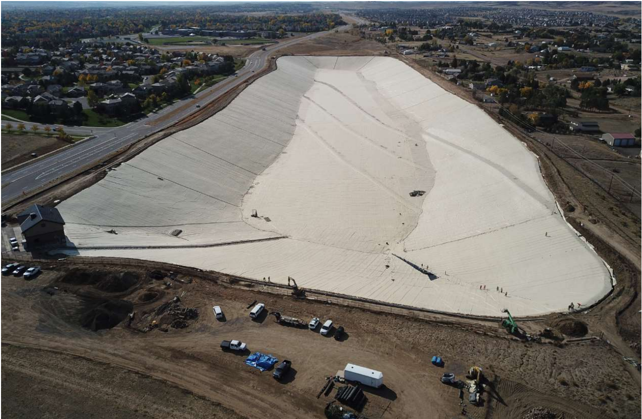
Chambers Reservoir Liner Under Construction
