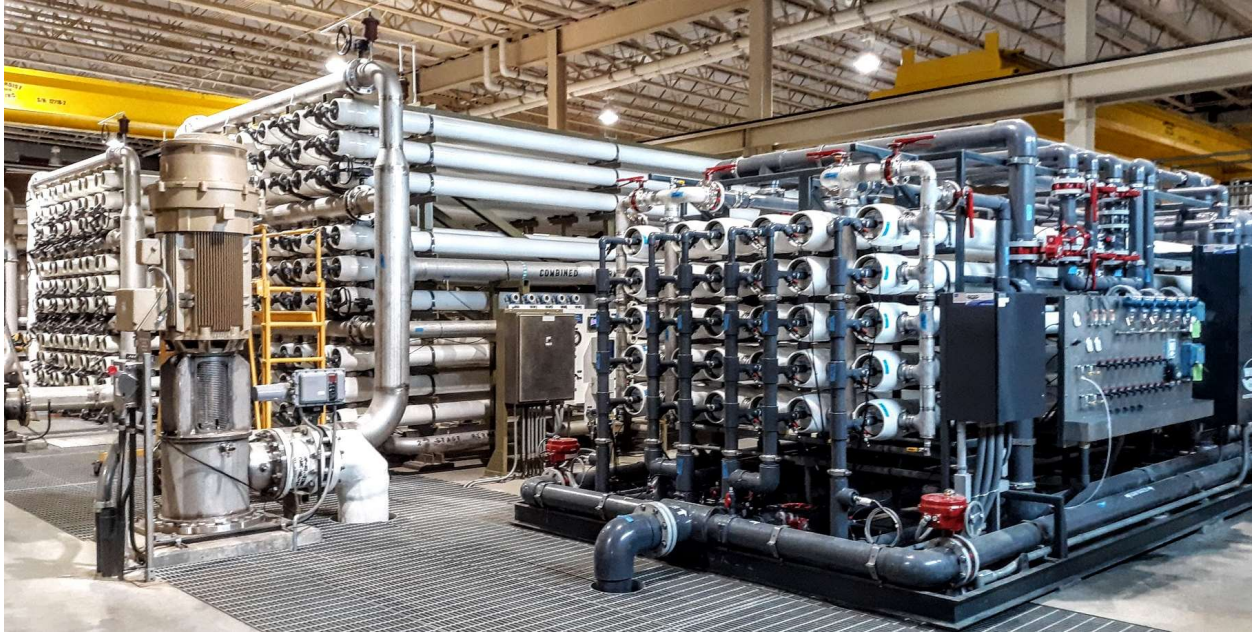
New RO Units for Water Production - JWPP
