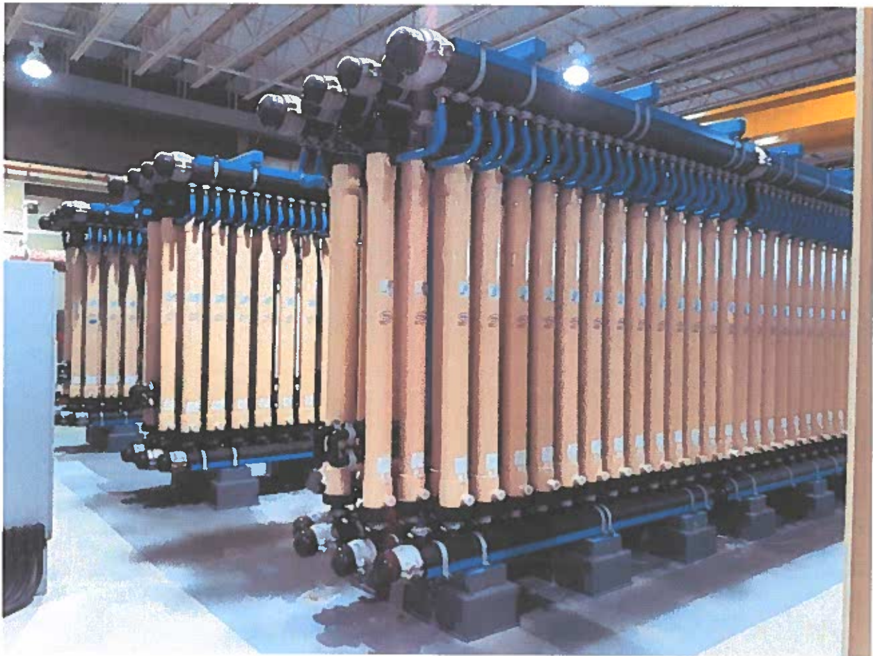
Pictured above are the RO membrane racks at the newly-reconfigured Joint Water Purification Plant.
